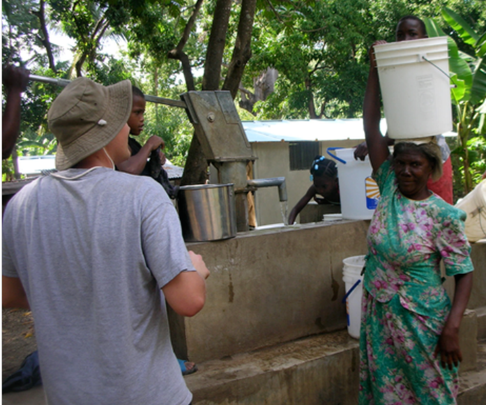
Figure 2 Existing hand pumped well in Lakoline Village
